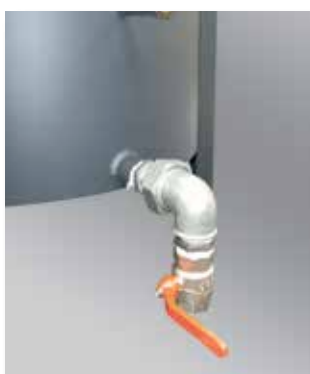
■ Manual discharge with ball valve
